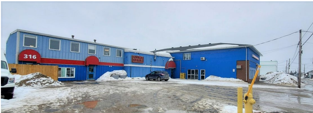
Figure 12 - 316 Spruce St. S in Timmins, new home of Living Space Shelter.
